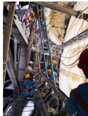
PMT module installing
